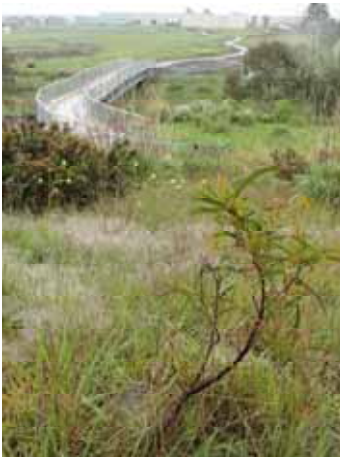
Bridge over Merri Creek
